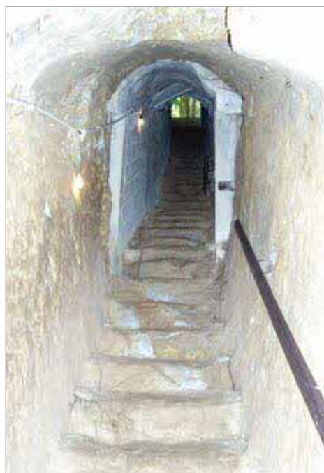
The stairs inside the Khao Nam Khang tunnel which was used as an escape route. Photo courtesy of Mahani Awang.
